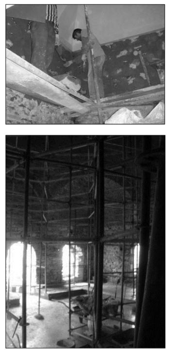
Fig. 8 Repairing of jointing
